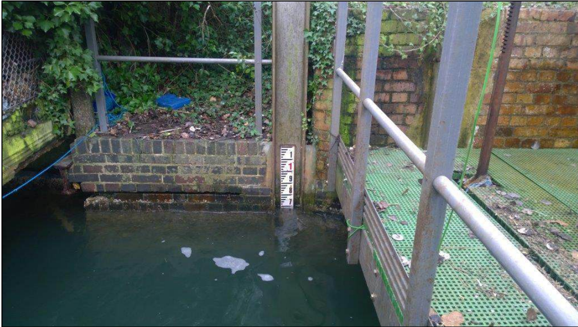
Figure 6.2 Gauge board installed in the Lagoon adjacent to the sluice gate. Photo taken at lake full water level.
